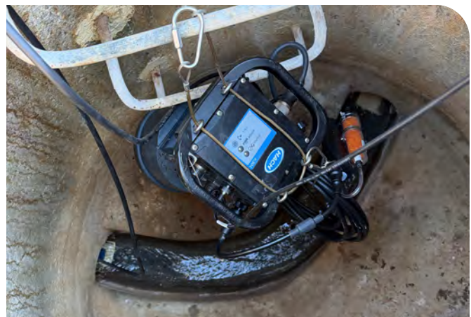
Figure 1. Photos provided by K-Flow. LEFT: Confined space entry for large diameter flow meter installation. RIGHT: Example of flow meter installation for sewer monitoring.
