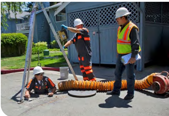
Figure 1. Photos provided by K-Flow. LEFT: Confined space entry for large diameter flow meter installation. RIGHT: Example of flow meter installation for sewer monitoring.
