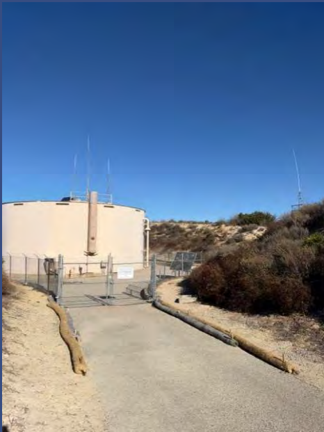
Tank and Pump Station Erosion Control
