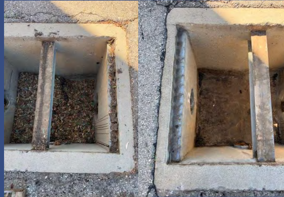
Clearing Catch basins at Tanks and Pump Stations
