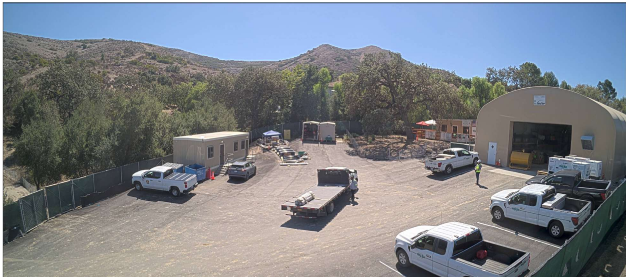
Laydown yard with temporary paving
