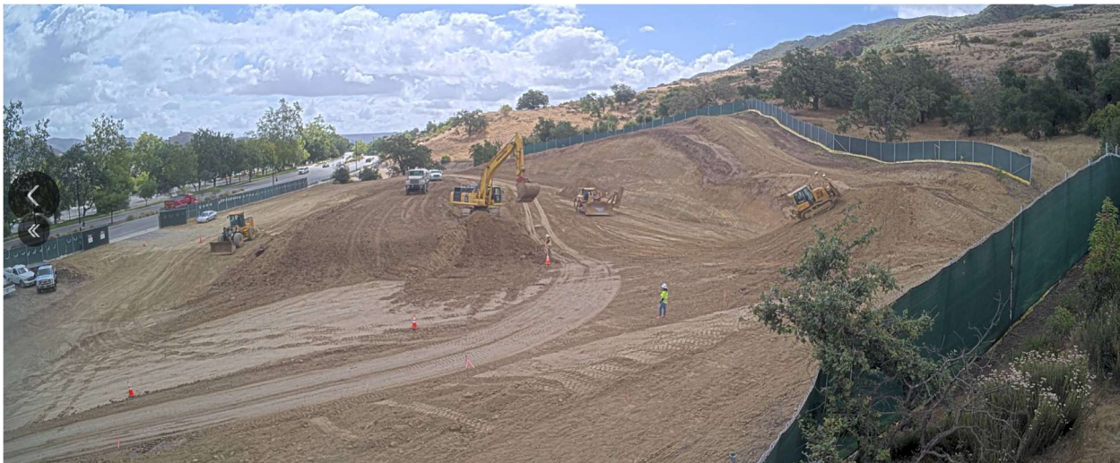
Mass Grading of AWPf site
