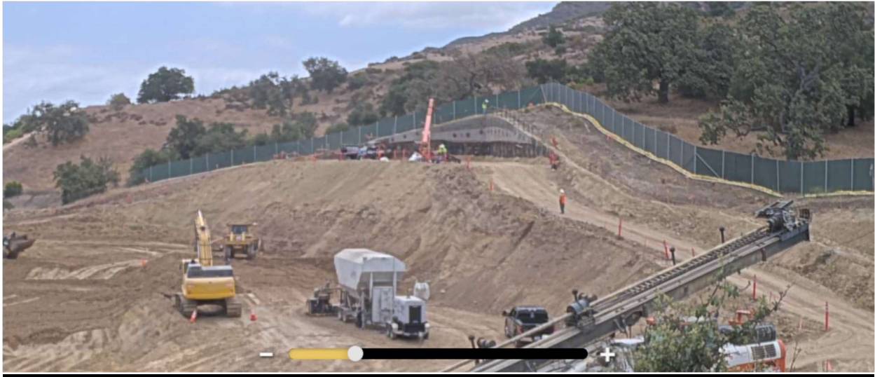
Soil Nail Wall Early Construction
